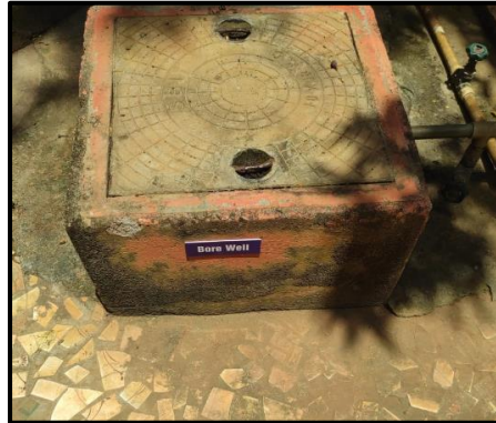
Water Management Activities observed in the campus
